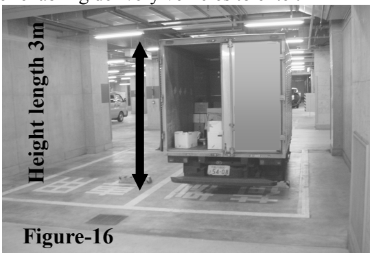
Figure 16. Example of loading space envisioned for 4-ton class delivery vehicle
