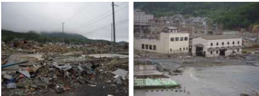
Near the earthquake center
