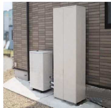
Fig.4 Home small heat & power generation
