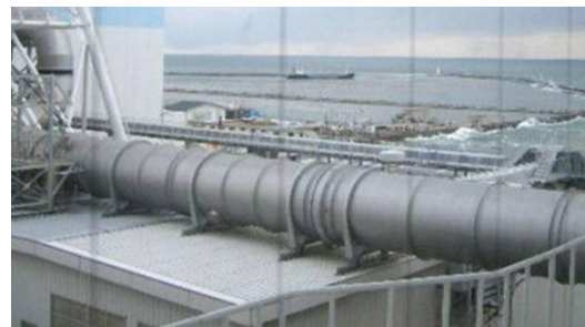
Fig.11 Ship taking refuge from Tsunami in Fukushima nuclear power plant.
