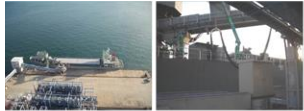
Fig.10 Electric supply wire and equipment.
